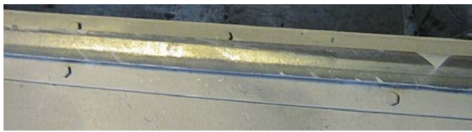
Fig. 3. Railway without channel – the contact surface is only the shiny one.
